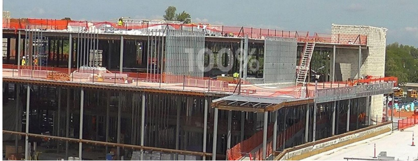
Exterior Framing South
