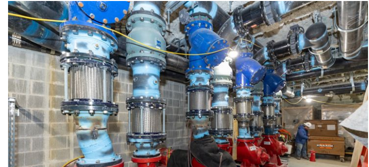
Mechanical Equipment Installation
