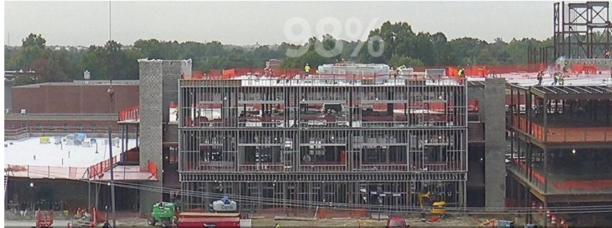
Exterior Framing North
