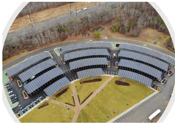
Bowie State University solar canopy parking lot.
